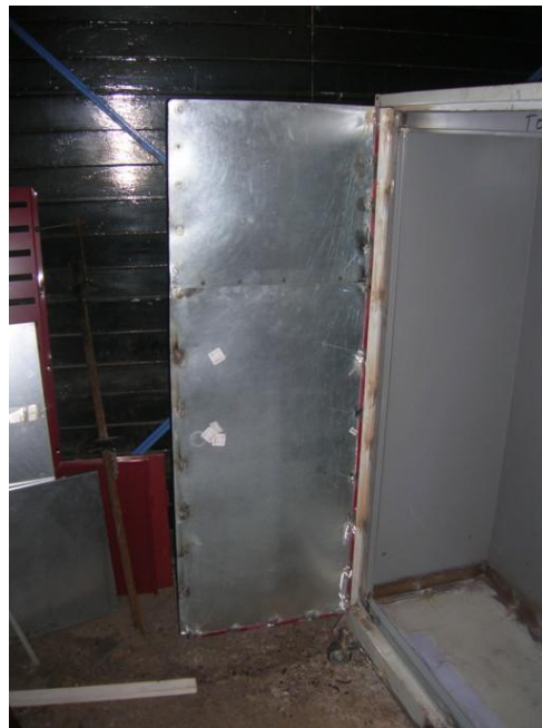
The doors insulated and skinned
