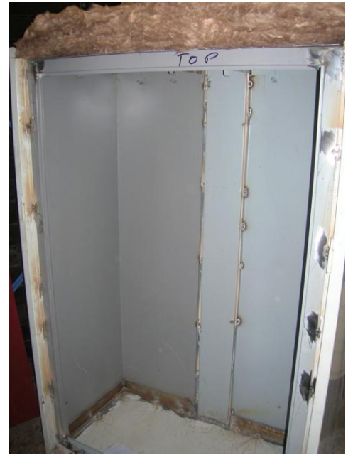
The remains of the 2 lockers welded in place with the infill
