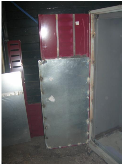
The galvanised shelves used as the Inner door skin, insulation packed in between
