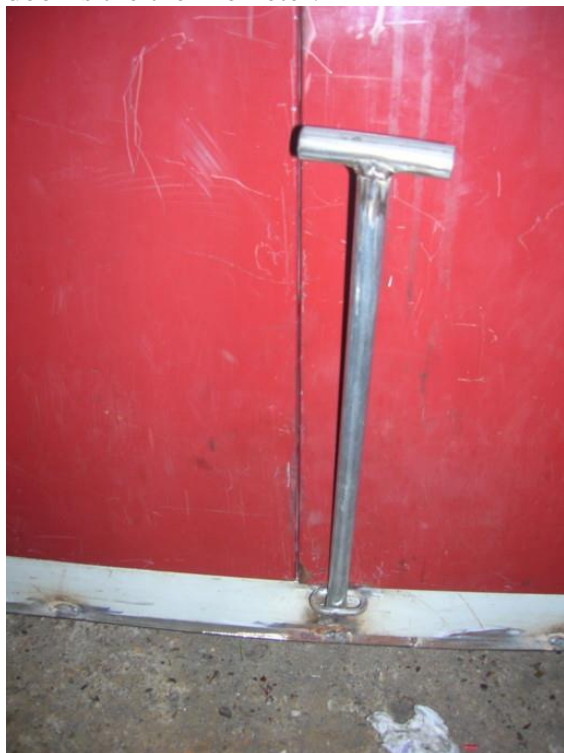
A chain link and tapered metal tube as the door closer, I know..... but it works!
